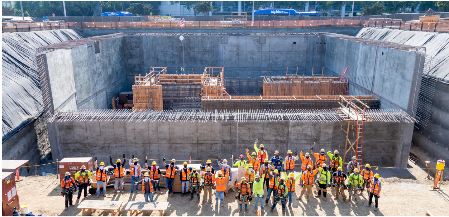
Kiewit's workforce on the project peaked at 13 staff and nearly 70 trade craft employees. Subcontractors brought the total craft workforce to nearly 100.
