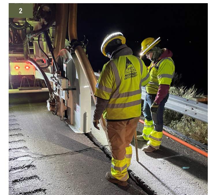
1. Two CleanFast trucks were purchased to support this project and diversify Kiewit’s capabilities. 2. The southern segment of the project required work during night closures. Reflective personal protective equipment and halo lighting on the crew’s hardhats was utilized to improve visibility.
