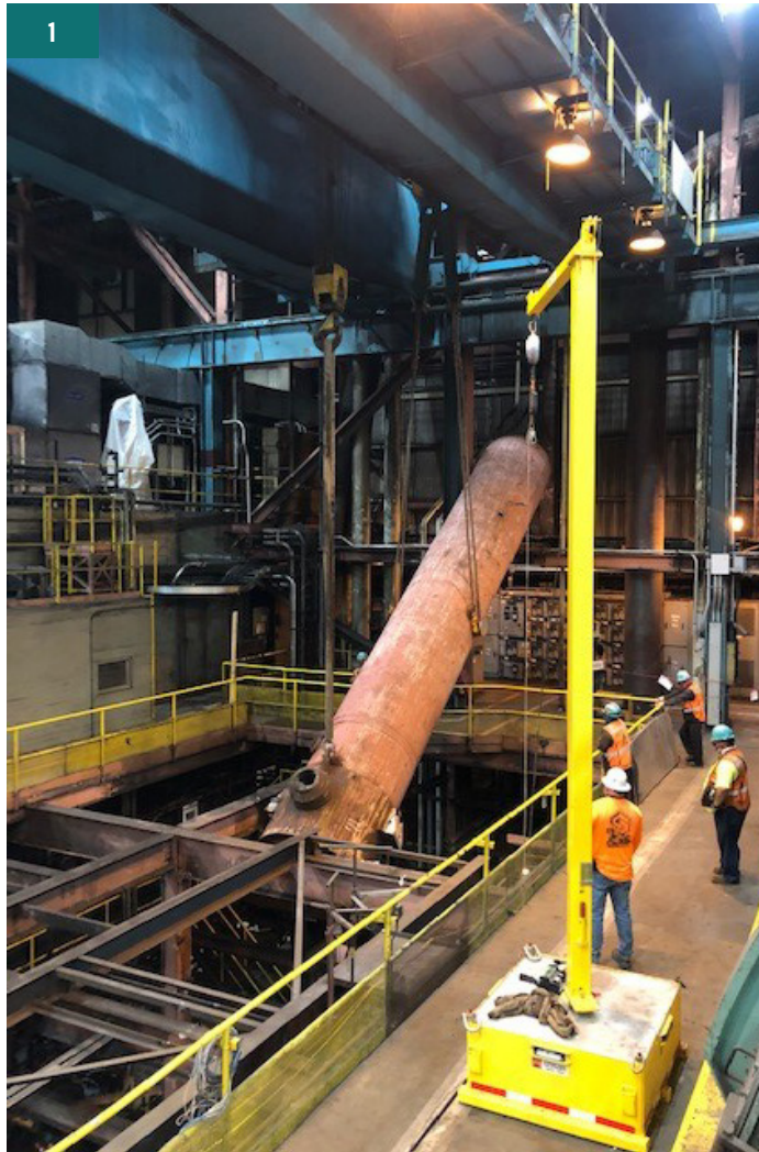
1. Crews remove an old feed water heater as part of the demolition work needed to prepare Unit 1 for new equipment. 2. Cranes were used to place sections of the 2,500-linear-foot of pipe rack in place over a canal.
