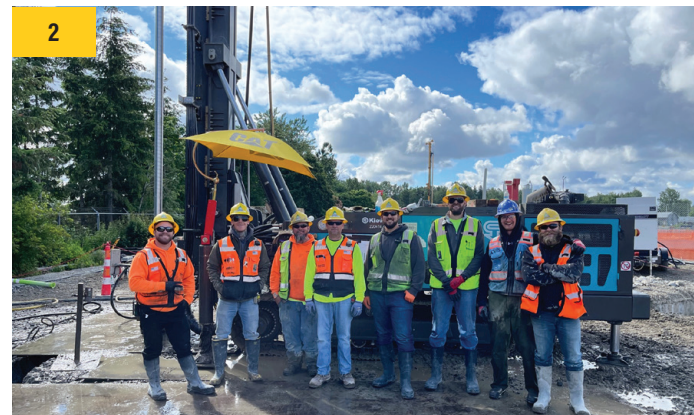
1. The soil mixing and jet grouting combination batching plant set-up. 2. The Columbia Boulevard team included experience staff and craft from across the company to provide in-house expertise to the project.
