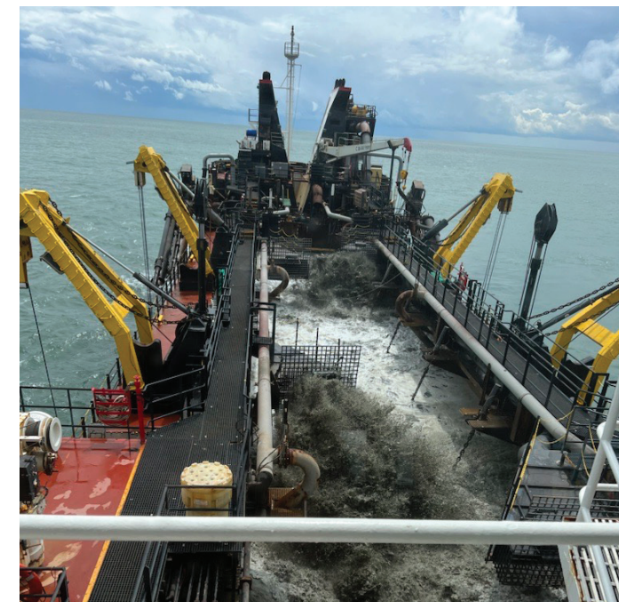
Weeks' crews work to restore a beach off the Delaware coast.
