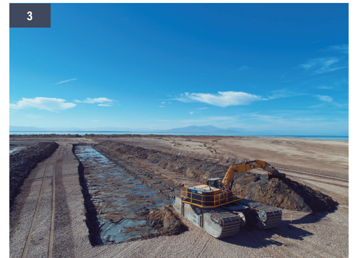
1. More than 150 pieces of equipment were used to complete work on the Species Conservation Habitat Project. 2. Crews built a new diversion structure, which diverts water from the New River to mixing basins, where it is mixed with water that's pumped from the Salton Sea before entering the habitat's ponds. 3. The scope of the project included installing nearly 3 miles of 30-inch high-density polyethylene (HDPE) pipeline.
