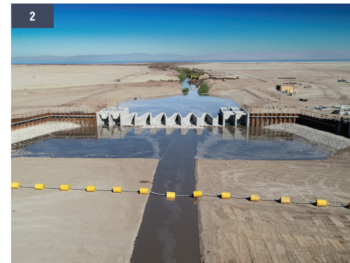
1. More than 150 pieces of equipment were used to complete work on the Species Conservation Habitat Project. 2. Crews built a new diversion structure, which diverts water from the New River to mixing basins, where it is mixed with water that's pumped from the Salton Sea before entering the habitat's ponds. 3. The scope of the project included installing nearly 3 miles of 30-inch high-density polyethylene (HDPE) pipeline.
